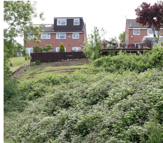
South West part of the site
